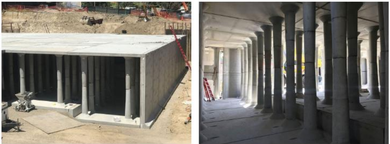
Figure 9 StormPrism System- example of proposed Infiltration Gallery
