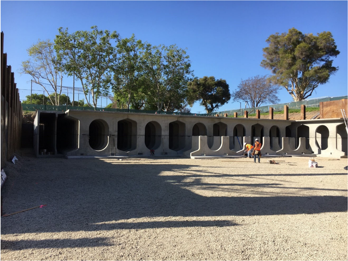
Figure 15. Example StormTrap installation at Bolivar Park in Lakewood, CA
